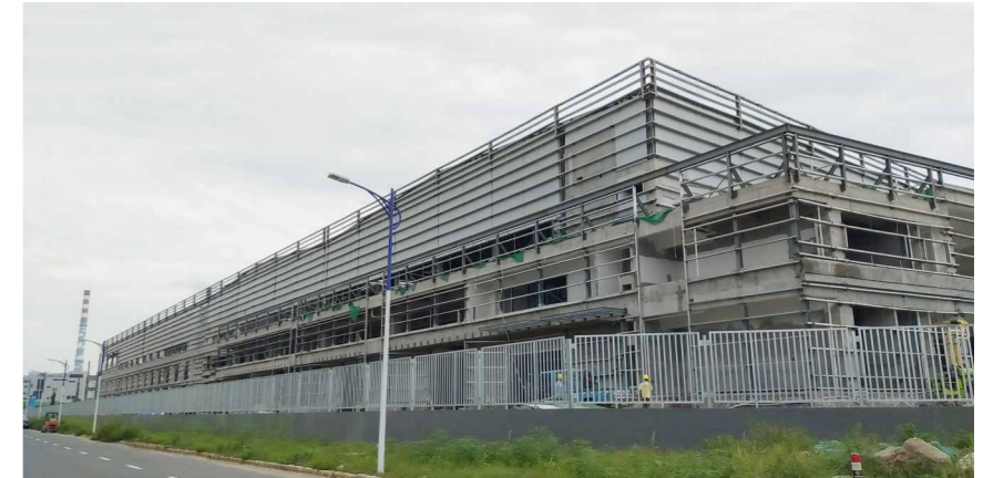
■ YIZUMI China Wusha Factory 3 is under construction
