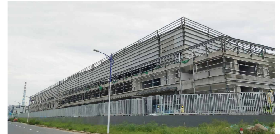
■ YIZUMI China Wusha Factory 3 is under construction
